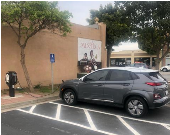
FIGURE 35: LEVEL 2 EVSE IN DOWNTOWN GUADALUPE (PHOTO: PLUGSHARE)
