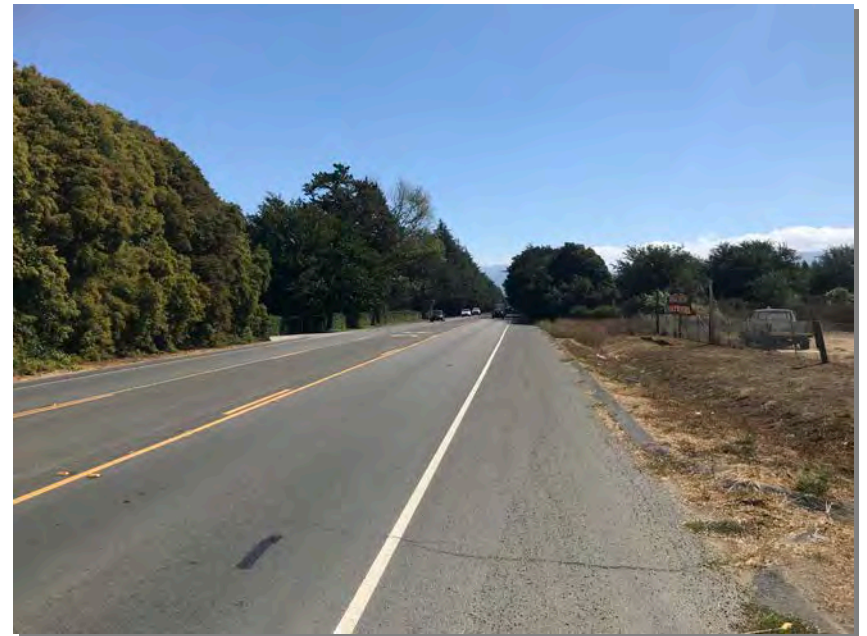
SR 246 outside of Buellton typically has highway shoulders, but they are not Class II bike lanes. Additionally, cyclists are often asked to share the road with traffic travelling in excess of 55 miles per hour.
