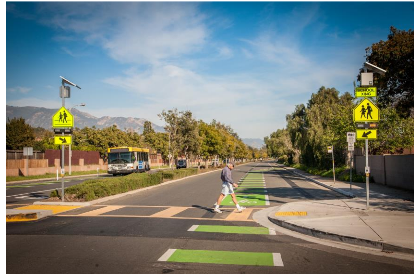
This intersection in Goleta includes many pedestrian safety features, including a flashing beacon, curb bump outs, a pedestrian refuge, and a high-visibility crosswalk.
