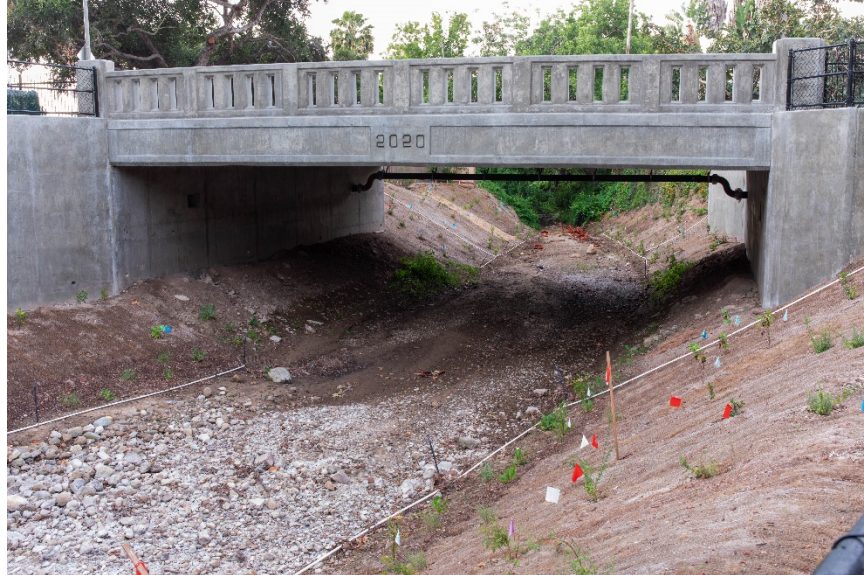
Figure 2 Quinientos Bridge Profile After
